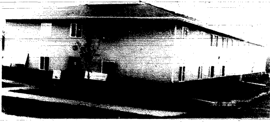
The 16-unit apartment complex, located on West 13th Street, will be available Oct. 1 for qualified tenants. The complex was developed by Carhart Lumber Company, Carhart family members and Wayne Community Housing Development Corporation.
